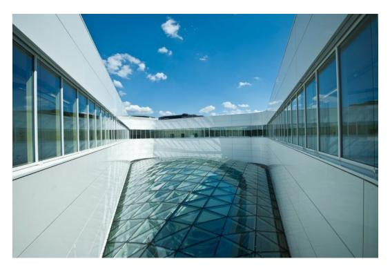
At about mid-height, a triangular skylight spans the whole of the atrium, its glass roof being a biaxially-arched lattice structure.
